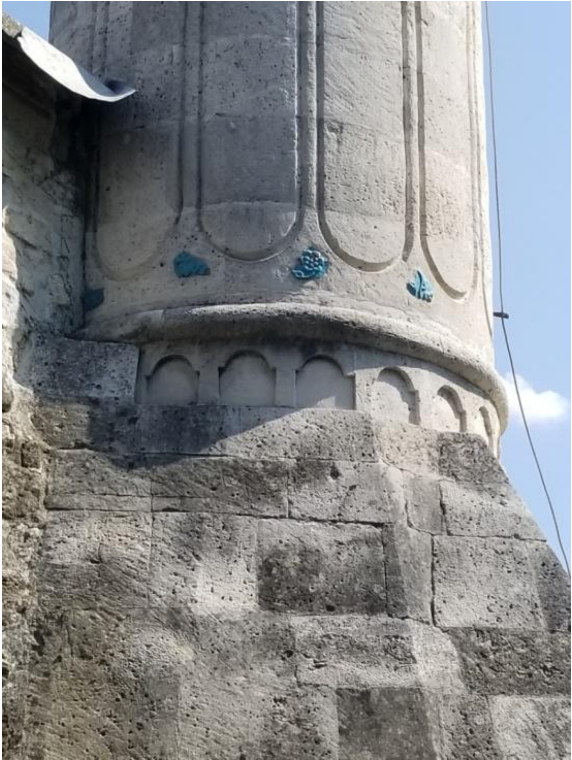
Fig. S1e: View of the glazed tiles on Yeşilce Mosque minaret.
