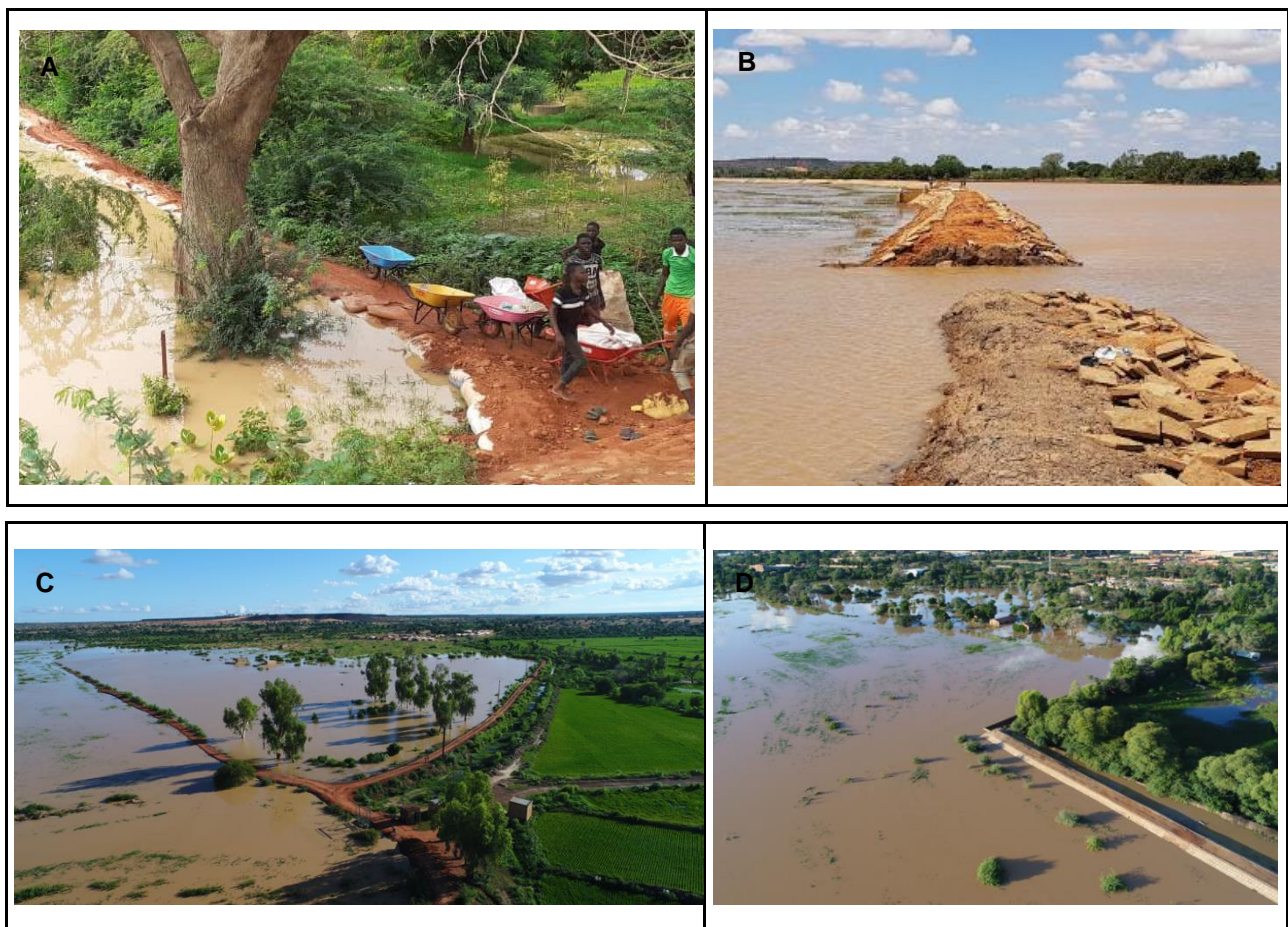
Figure 7. The Niamey levees during the 2019 and 2020 flood events: (A)(top-left) the bridges levee (sector B) raise with sandbags on 18/8/20 ( h = 651 cm), (B)(top-right) the levee break in Lamordé (Sector A) on 6/9/20 ( h = 679 cm), (C)(bottom-left) aerial view of Kirkissoie levee on 30/8/19 ( h = 619 cm), (D)(bottom-right) aerial view of Saga levee on 30/8/19 ( h = 619 cm).
