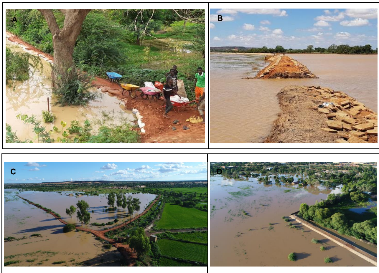
Figure 7. The Niamey levees during the 2019 and 2020 flood events: (A)(top-left) the bridges levee (sector B) raise with sandbags on 18/8/20 ( h = 651 cm), (B)(top-right) the levee break in Lamordé (Sector A) on 6/9/20 ( h = 679 cm), (C)(bottom-left) aerial view of Kirkissoie levee on 30/8/19 ( h = 619 cm), (D)(bottom-right) aerial view of Saga levee on 30/8/19 ( h = 619 cm).
