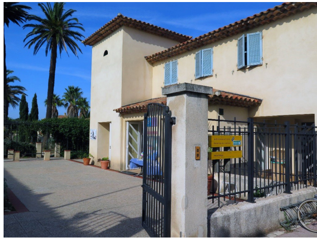
Fig. 8. – In the background, the ‘bats tower’ (Tour du Palmier) in the village of Porquerolles. The half-moon opening at the top of the tower is the entrance to the shelter specially built to house a colony of Geoffroy’s bat Myotis emarginatus . Photo © Charles-François Boudouresque.
