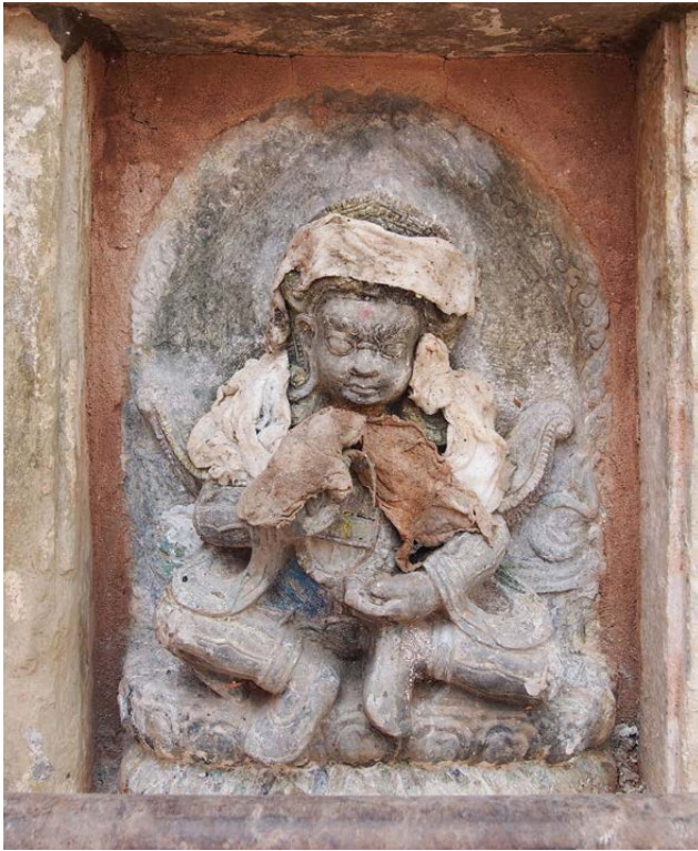
CLEANING OF THE DHRTARASTRA SCULPTURE Located in the central niche of level 1 facing south. © UNESCO | T. Schrom | Jul 3, 2017
