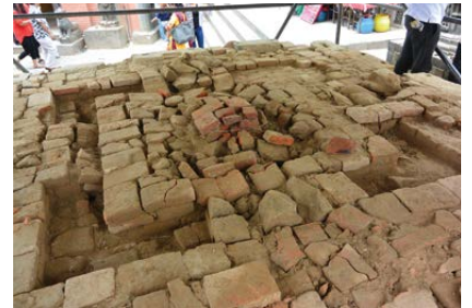
VIEW WITH THE CENTRAL SHAFT REMOVED View from the east © UNESCO | D. Andolfatto | Aug 30, 2016
