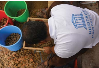
SORTING TSHA TSHAS Following the removal of the miniature stupas from the rubble and the four L-shaped voids they were sorted according to size and type. © UNESCO | D. Andolfatto | Aug 22, 2016
