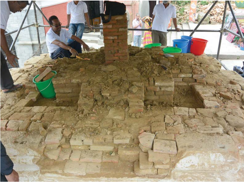
THE CENTRAL SHAFT AND L-SHAPED VOIDS View from the east © UNESCO | D. Andolfatto | Aug 29, 2016
