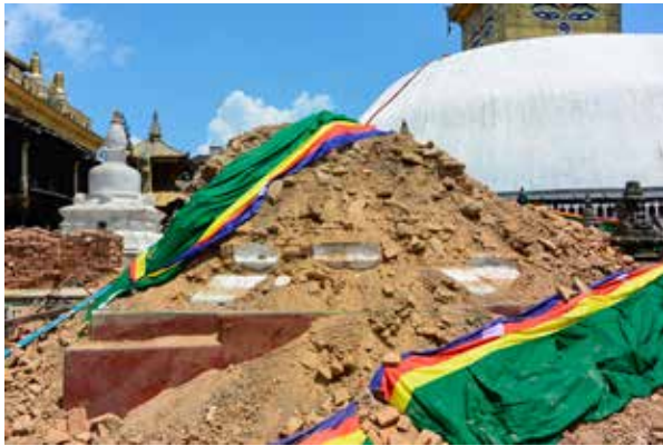
Fig 7. Tashi Gomang Stūpa shortly after its collapse. 1 st May 2015. © D. Andolfatto/UNESCO Kathmandu
