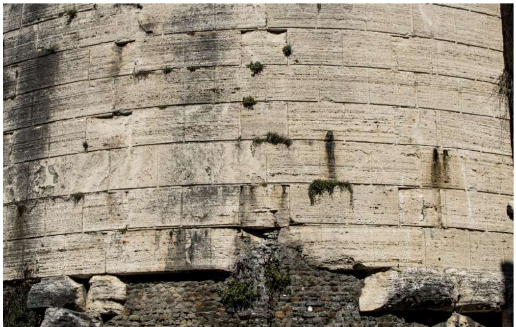
Fig. 02. Detail photo of travertine blocks treated as a fake ashlar. (photo by the author).
