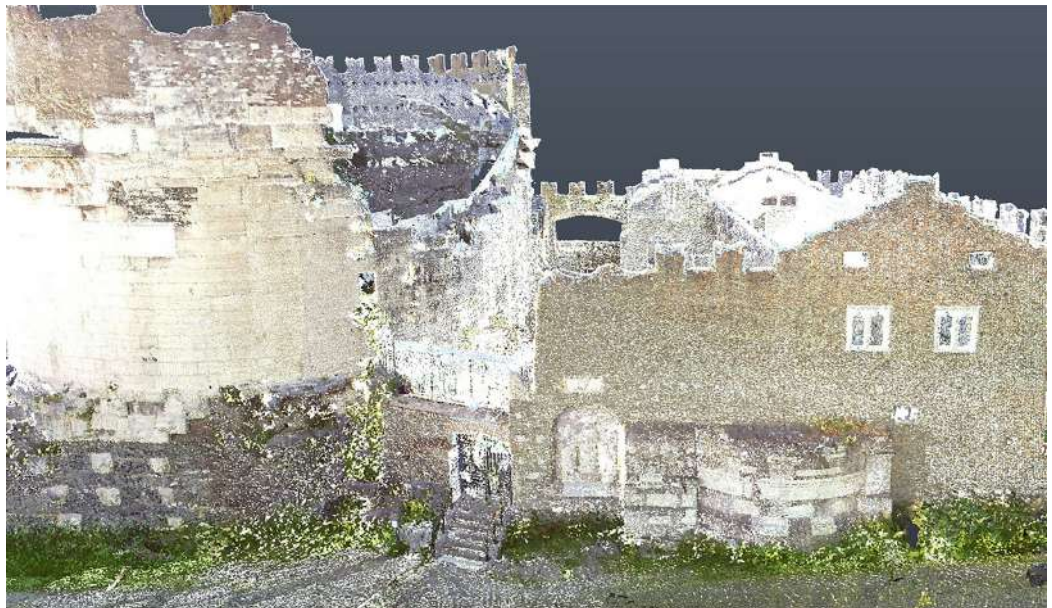
Fig. 06. Point cloud with RGB values of the monumental complex of Cecilia Metella and the castrum Caetani. (Elaboration by the author).
