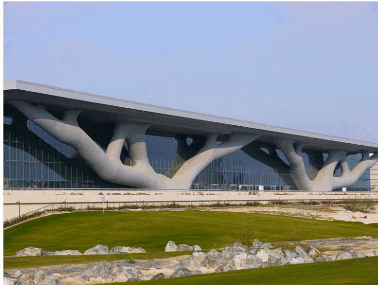
Figure 3.10: Qatar National Convention Center, by architect Arata Isozaki in Doha, Qatar, exhibiting organic truss-shaped pillars.
