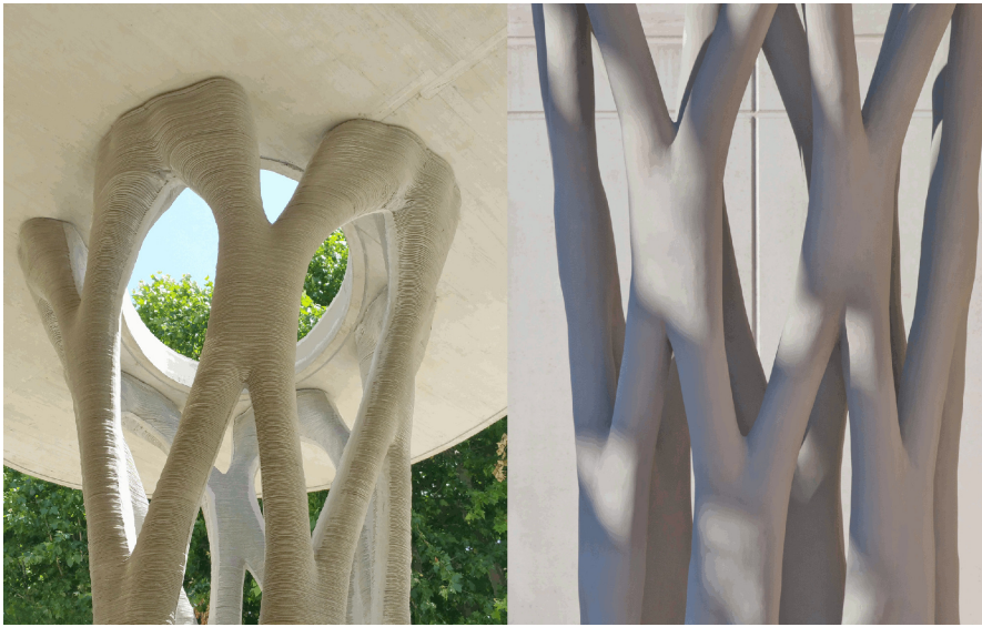
Figure 3.9: Before (left) and after (right, photo by Lisa Ricciotti) surface smoothing obtained through manual coating.
